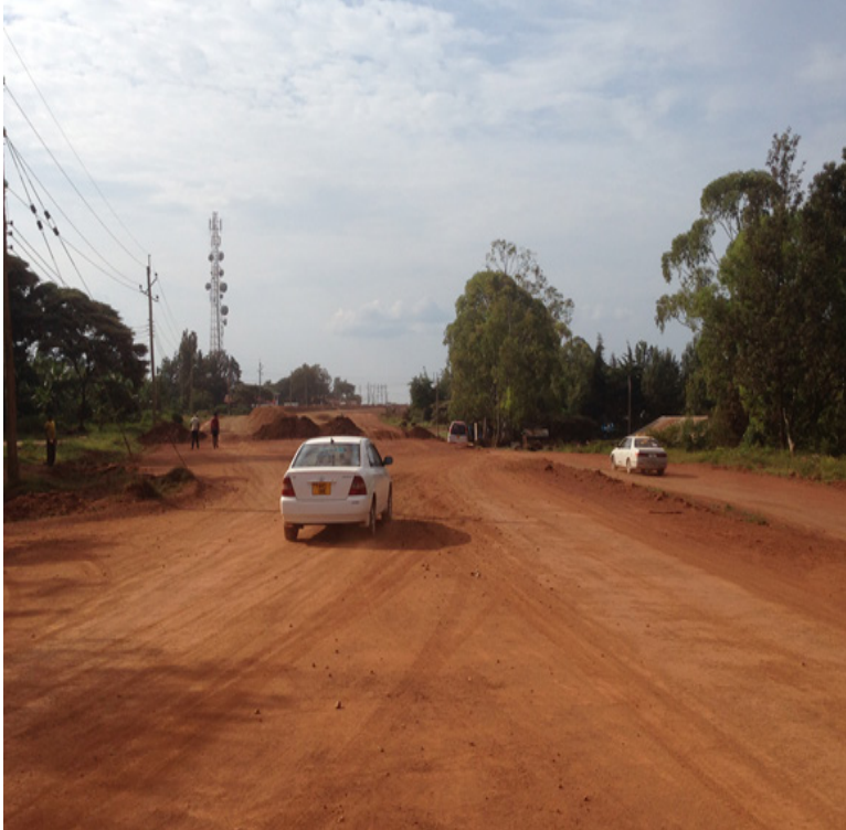
Figure 3. Local Road Construction in Kayanga, Tanzania
